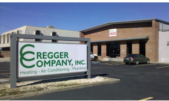
With 28 branches across several states, 31-year-old Cregger Company expands a commitment to its air conditioning and heating business
